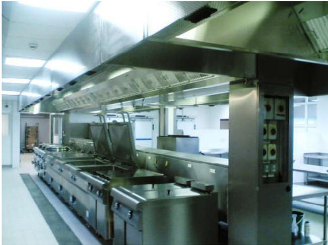
Specialist Ventilation Services range of high efficiency kitchen ventilation canopies are designed with low energy consumption in mind. Not only in everyday use but also in our manufacturing processes where welding is kept to a minimum using state of the art bonding materials specifically developed for stainless steel construction where hygiene is important.
